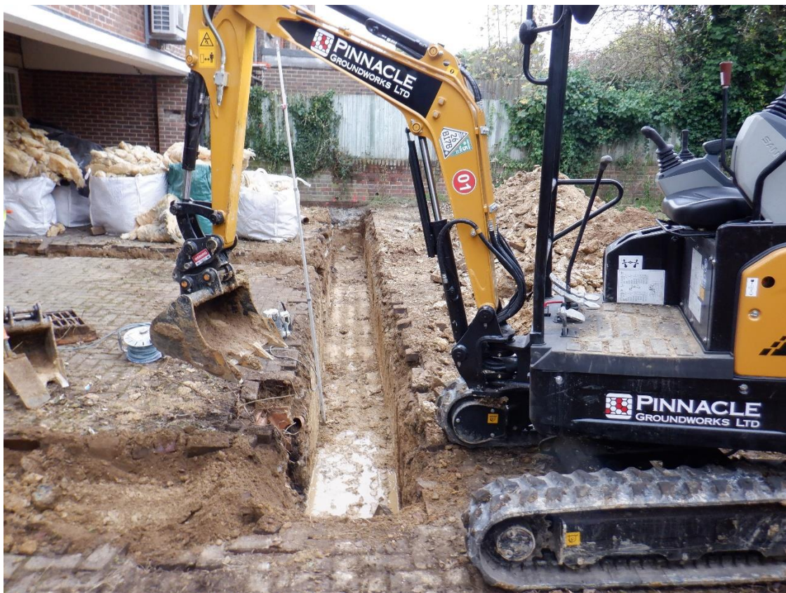
Plate 3. Foundation trenching (looking North)
