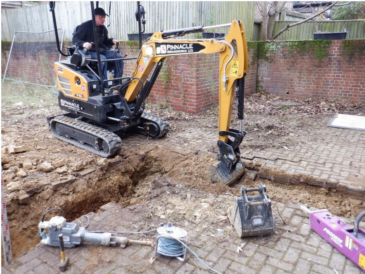
Plate 1. Initial foundation trenching (looking South)
